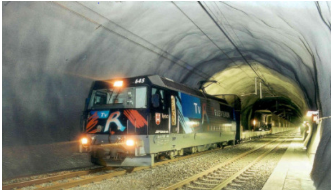
Figure 9: The Vereina tunnel in operation
