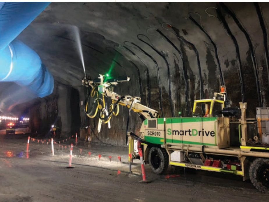
Above, figure 4: SMART DRIVE electrically- powered spraying robot PHOTO: NORMET
